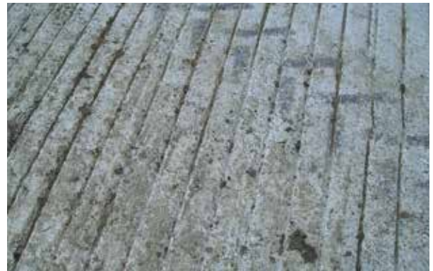
Textured concrete, more traction without slipping
