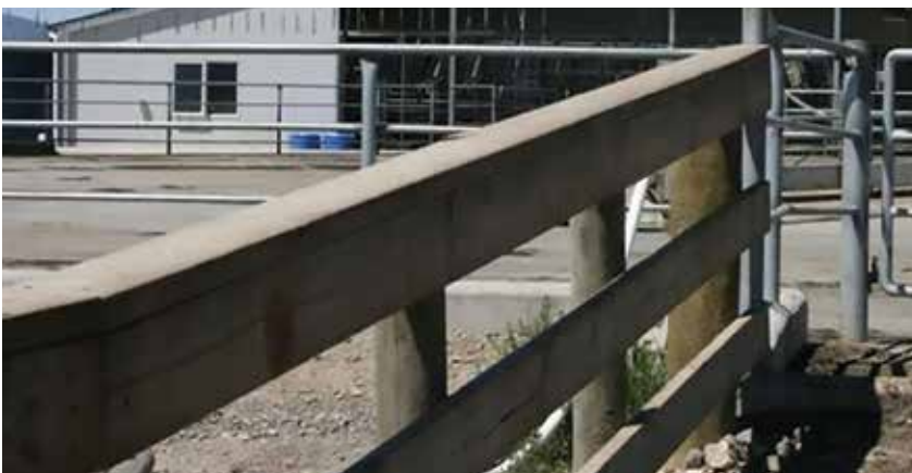
Wooden railings leading to the yard entry provide a strong visual barrier and are comfortable for cows to brush up against.
