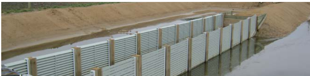
Sludge bed with double weeping wall and PVC battens.
