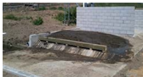
Concrete pad for dewatering stone trap solids.
