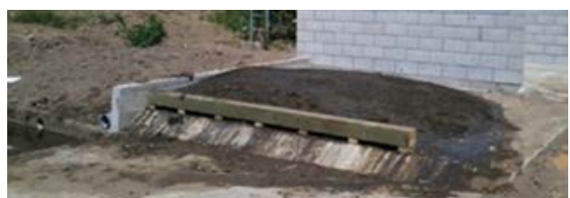
De-watering pads and solids storage bunkers
