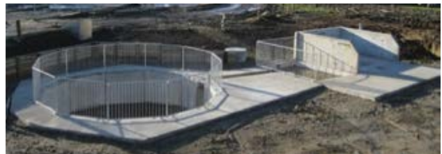
Sand traps and sumps
