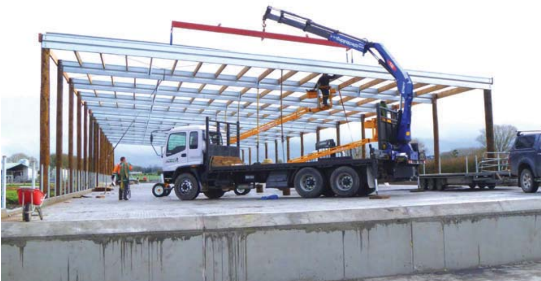
Building frame construction
