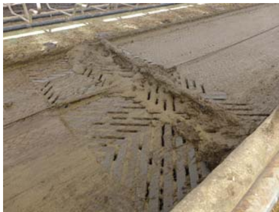
Slatted covers over a cross-collection channel for scraped dairy effluent
