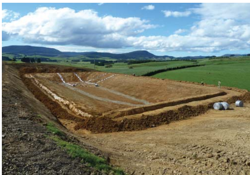
Effluent pond under construction
