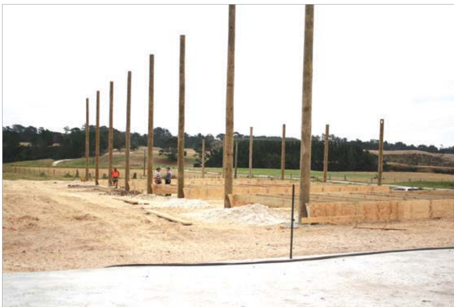
Timber pole structure
