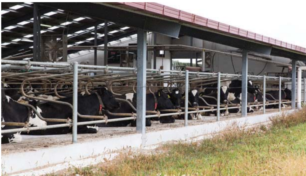
Open sided structure (Note: internal fans)
