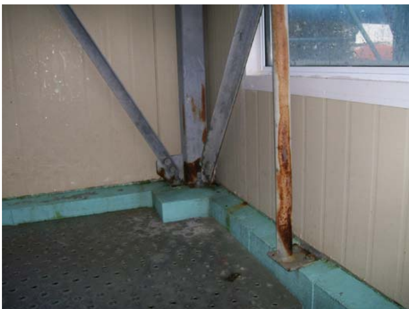
Steel corrosion
