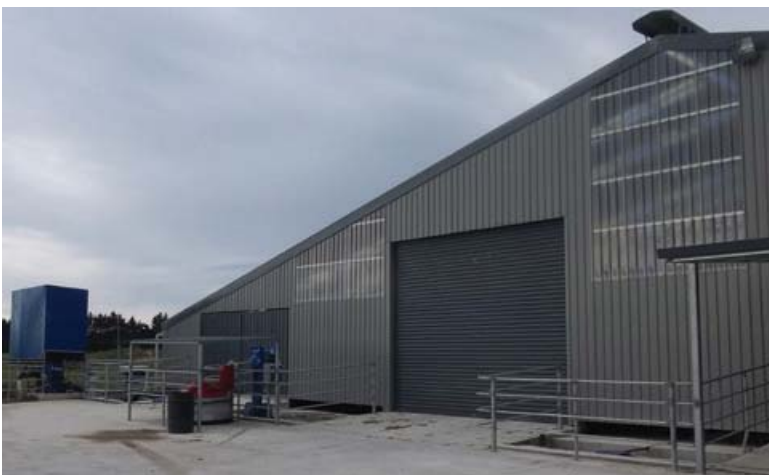
Effluent pit and pump
