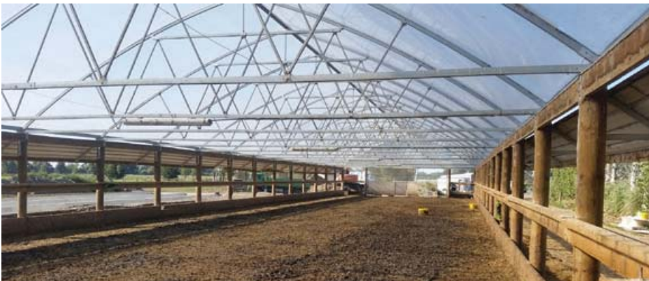
Plastic (clear PVC) roof
