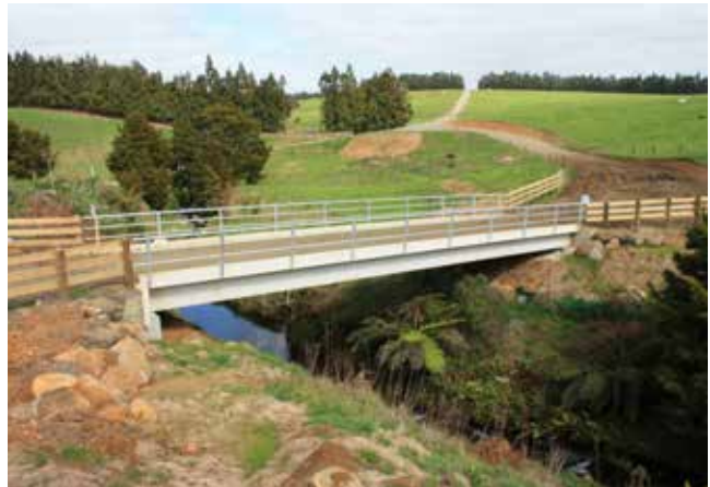
A well-constructed crossing.
